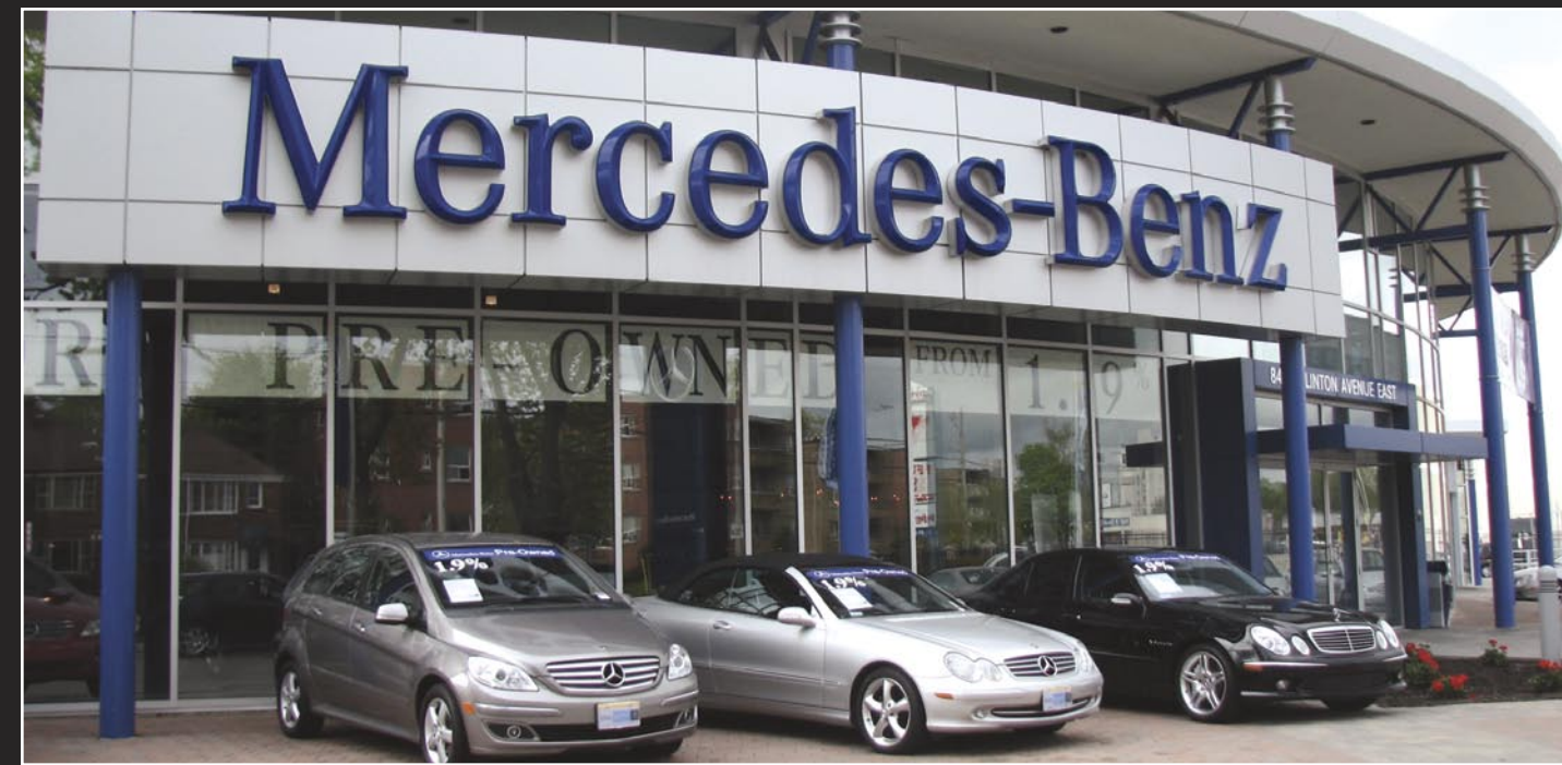
FEATURES – Curtain Wall | Aluminum Composite Panels | Interior Glazing LOCATION – Midtown Dealership | Toronto ON
