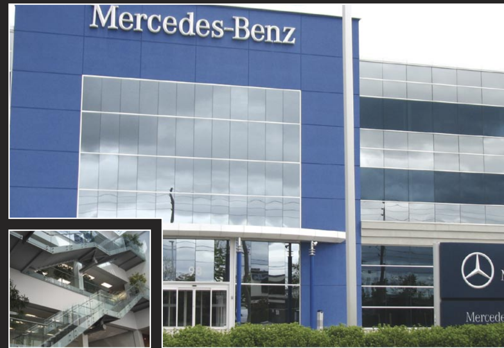
FEATURES – Curtain Wall | Aluminum Panels | Aluminum Column Covers | Skylight LOCATION – Canada Head Office | Toronto ON
